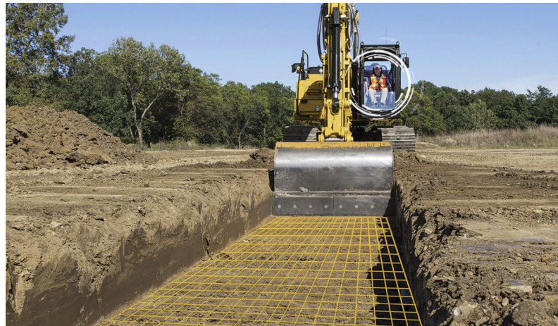
Figure 2. The grading operation using an excavator [10].
