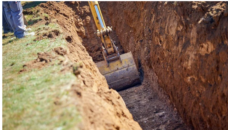
Figure 3. The trenching operation using an excavator [14].
