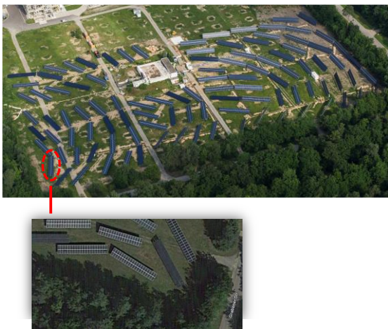
Figure 3. Solar park at the North Campus of the KIT with shaded array. The array has an inclination of 15° and orientation of 30° west.
