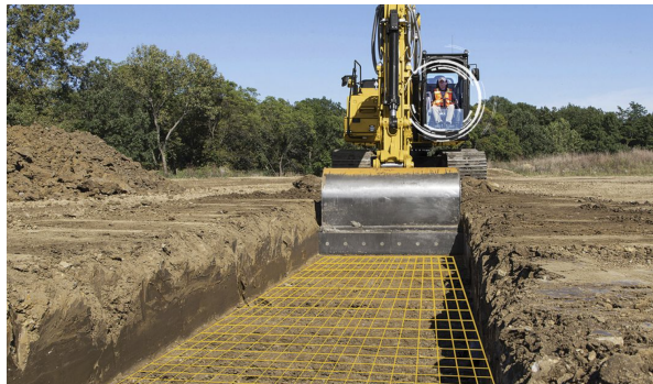
Figure 2: The grading operation using an excavator [9].
