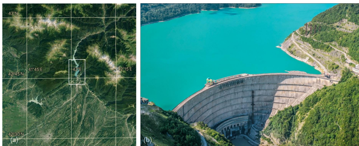
Figure 3.1: Enguri Dam presentation: (a) Satellite image mapped on the globe ©Google Earth. The white rectangle represents the localisation of the dam and the reservoir. (b) Aerial view of the Enguri Dam and its reservoir ©Georgia Travel Guide.
