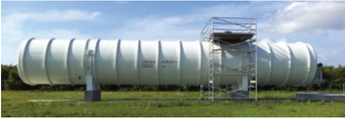
Figure 5.7: Photo of the LH 2 tank converted to a zero boil-off tank. Source: 13
