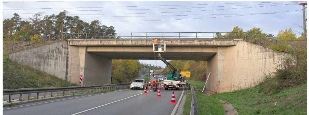
Figure 7. General view of concrete portal frame bridge 12842.
