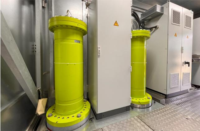
Figure 4: Picture of the Stornetic FESS with the two 60 kW flywheels.
