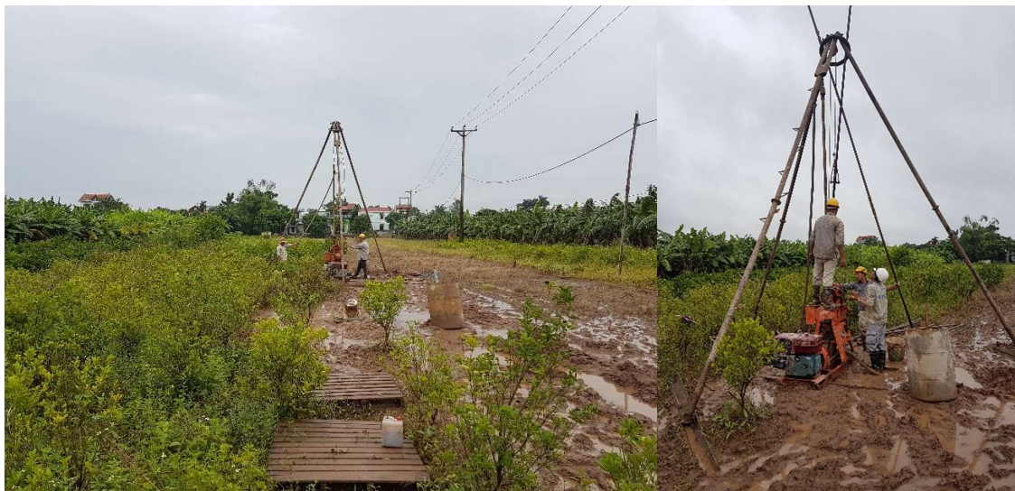
Figure 17: Rotary drilling in Van Phuc (RD42, 2017)
