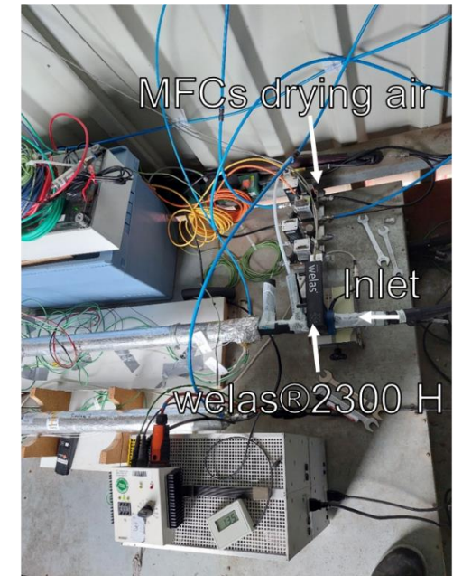
Top view of inlet
