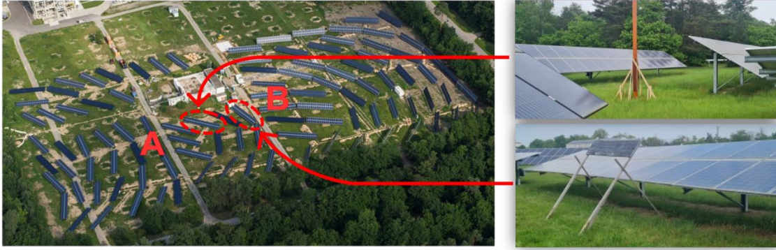
Figure 1. PV tables of the solar park on the north campus of the KIT. Selected PV tables for the investigation of shading are circled in red with their respective shading scenarios.
