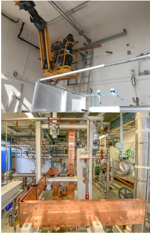
Figure 2: Installing the power supply for the test track
