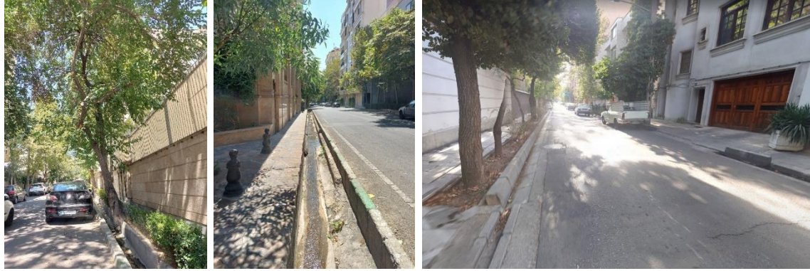
Figure 4.35. The pavement in the secondary streets in the Darrous Neighborhood (Author, 2022)
