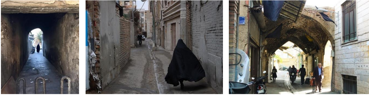
Figure 4.17. The construction quality in Sanglaj neighborhood (Amirhasani, 2017)
