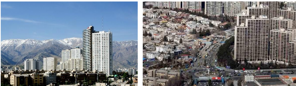
Figure 4.48. The quality of the buildings in the Shahrak-e Qarb Neighborhood (Zare, 2021b)
