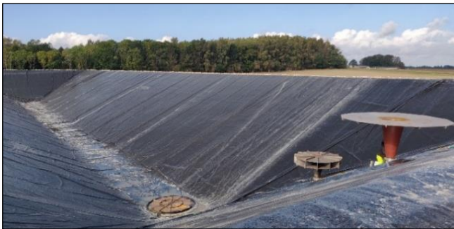
Figure 1: Diffuser installation.
