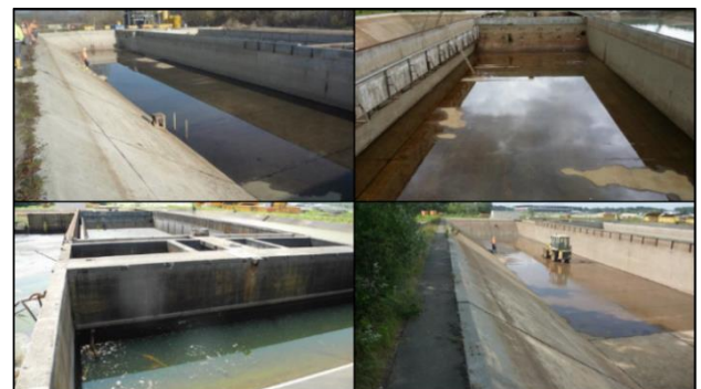
Figure 1: Multi-basin of infrastructures at the IN-Campus (Germany), pictured from different angles (Stettner and al. 2016).
