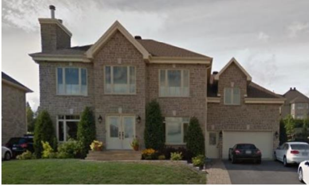
Figure 4: Front view of the experimental house No.1
