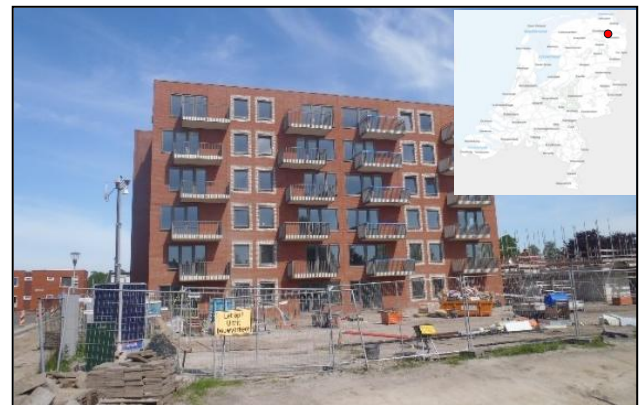
Figure 1: The Hoogezand pilot site apartment building, borehole heat exchanger field area in the foreground. (Location of Hoogezand within Netherlands indicated on map).
