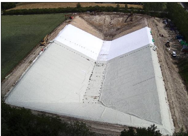
Figure 2: Liner installation.
