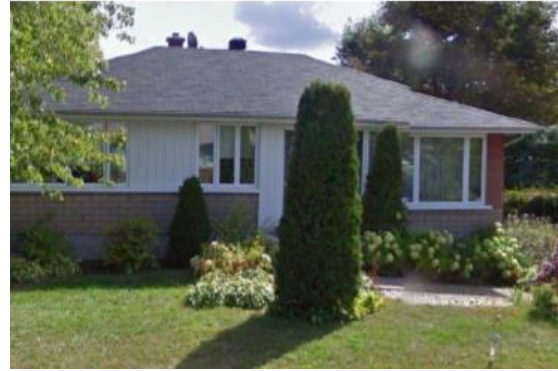
Figure 6: Front view of the experimental house No.2
