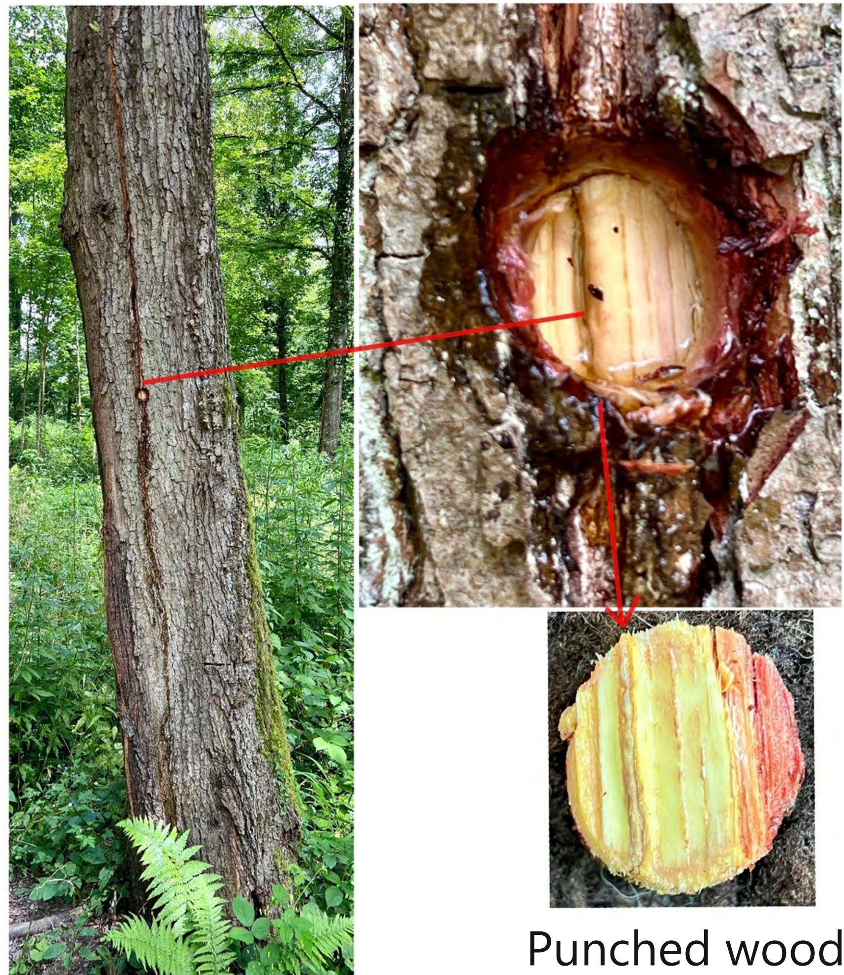
Crack behind growth strip next to older rib. Plenty of water leakage after punching!
