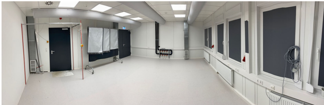
Fig. 251 Picture of concrete floor lab-space in the Innovation Village building
