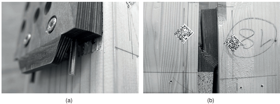
Figure 7.14: Imprint of milled surface in softwood (a) and failed connector (b).
