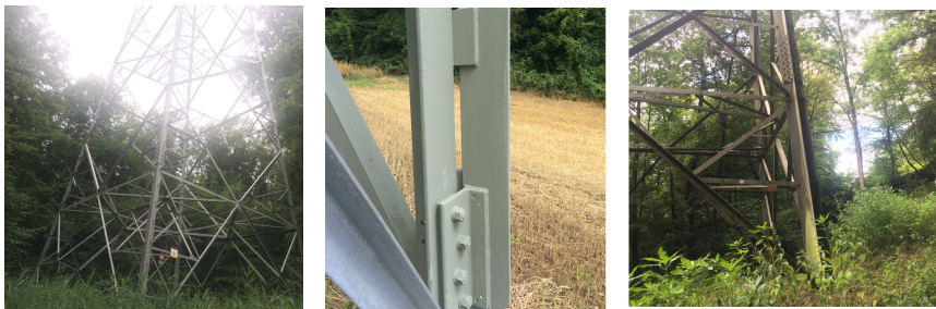
Figure 2.14: Visual depiction of predominant tower leg profiles suitable for installation: L-profile (left image), jointed X-profile (middle image), and standard X-profile (right image).
