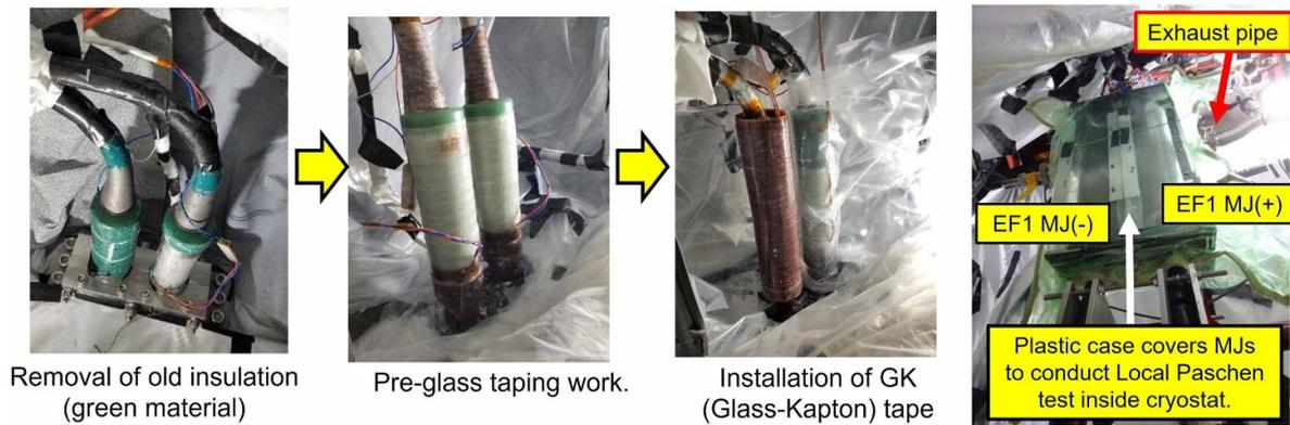
Figure 4. Insulation reinforcement work and local Paschen test.
