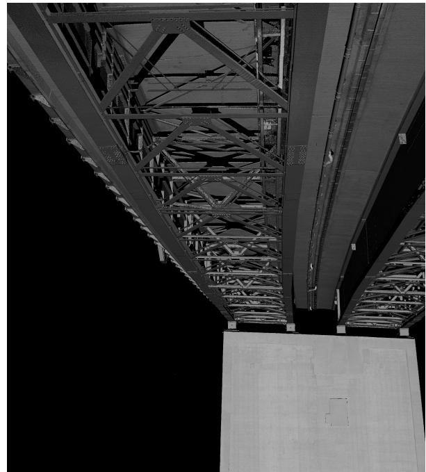
Figure 1. Extract from the 3D point cloud of span 7 of the motorway bridge. Intensity values are shown as grey scales.
