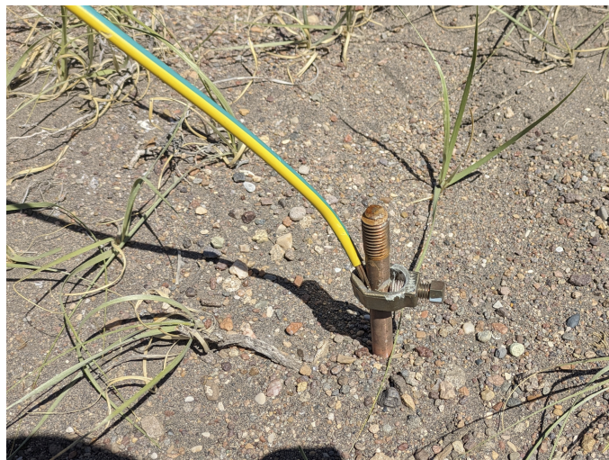
Figure A.4: Picture of the ground rod at LA with the clamp connecting the rod to the ground cable of the station.
