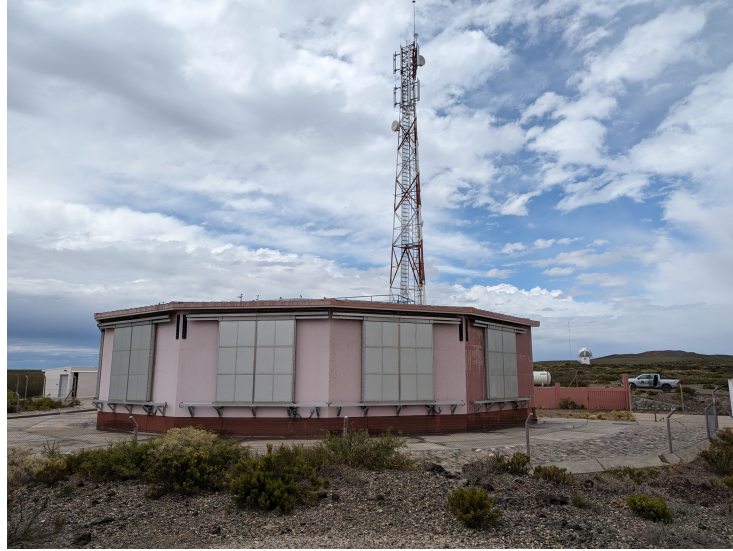
Figure 3.2: Fluorescence detector site Los Morados. The windows with closed shutters to four of the six telescopes are seen. Behind the FD building, a communication tower of the microwave link to the central campus is erected. In the back, a facility with a round roof can be seen that contains a LIDAR instrument. This particular LIDAR is not in operation anymore but LIDARs at Coihueco and Loma Amarilla still are.
