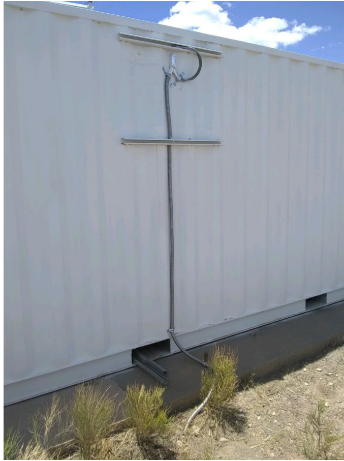
Figure A.3: Picture of the container at the CLF with the cable tube for the fiber cable to enter into the container.
