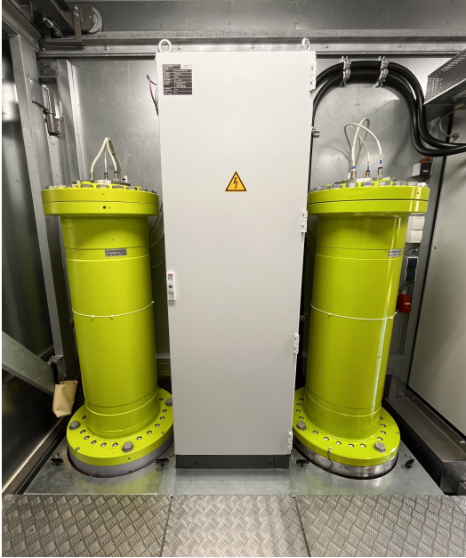
Fig. 6: Inside view of the container holding the two 60 kW Stornetic high-speed FESS.
