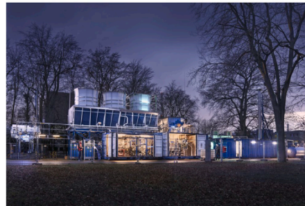
Fig. 5. The supercritical organic Rankine cycle MoNiKa (Modular Low Temperature Cycle Karlsruhe) at the Karlsruhe Institute for Technology (KIT). Left: Comparison of sub- and supercritical Rankine cycle, reproduced from [57] with permission given by Elsevier. Right: Photo of the facility, a 1 MW thermal supercritical ORC using propane as working fluid.
