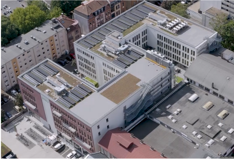
Figure 6.5: The 119 kWp PV plant with mixed east-west orientation at GCP no. 6.
