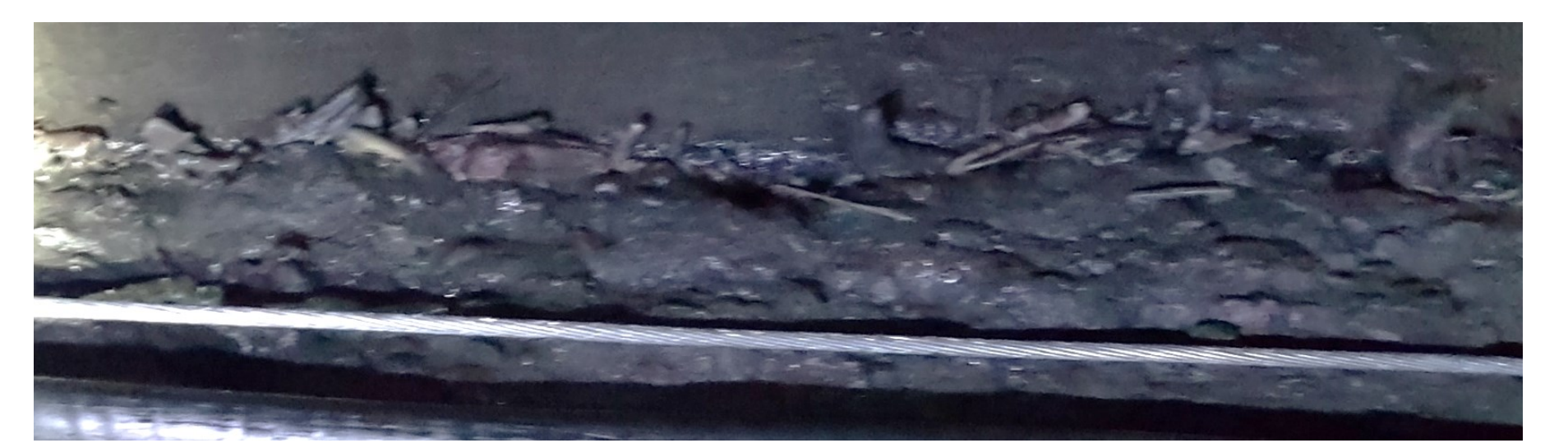
Part of a 40 m long open construction joint found at km 13.7 in the pressure tunnel. In this tunnel section, mud, larger fish and pieces of wood and plastic got stuck (Photo B. Aberle).
