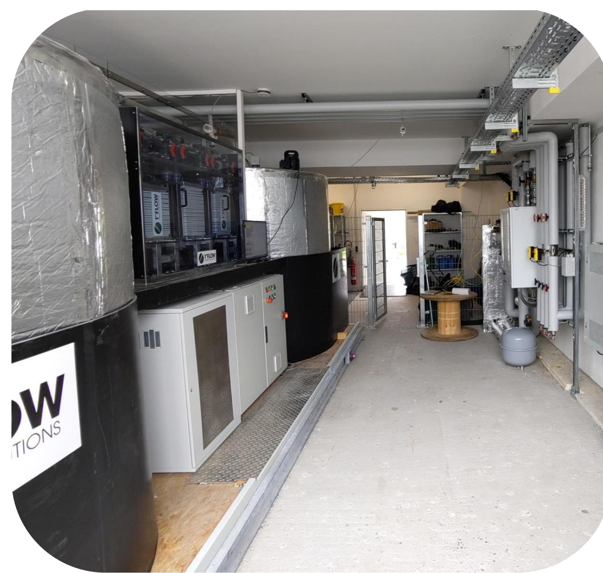
Fig 1. Installation in Bruchsal, Germany with the VFB (left) and TCM (right)
