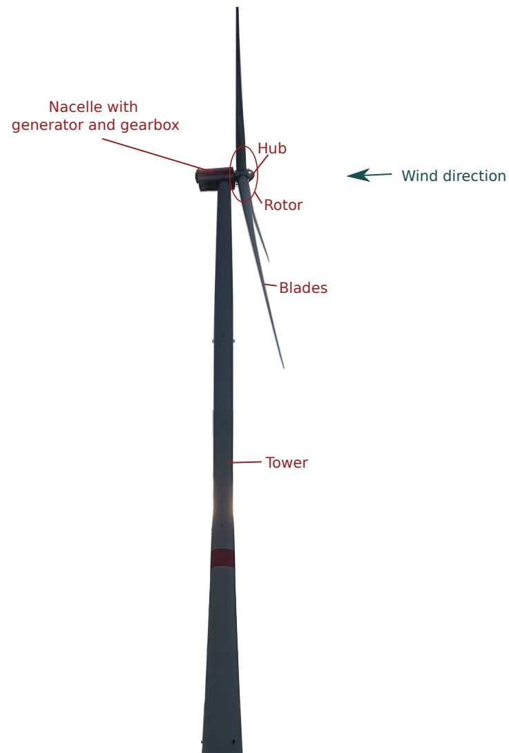
Figure 2.4: Northernmost WT of the WF Tegelberg, photographed by Laura Gaßner. The tower of an onshore WT is supported by a foundation, which is not shown in this figure. At the top of the tower is the nacelle, which is aligned in wind direction. Inside the nacelle is, amongst others, the generator, the gearbox, and the control system. Not highlighted in this illustration are the wind vane and the anemometer, which measure the wind speed and direction. The WT blades are attached to the front of the nacelle and face into the wind. They are held in position by the hub. The blades and the hub form the rotor.
