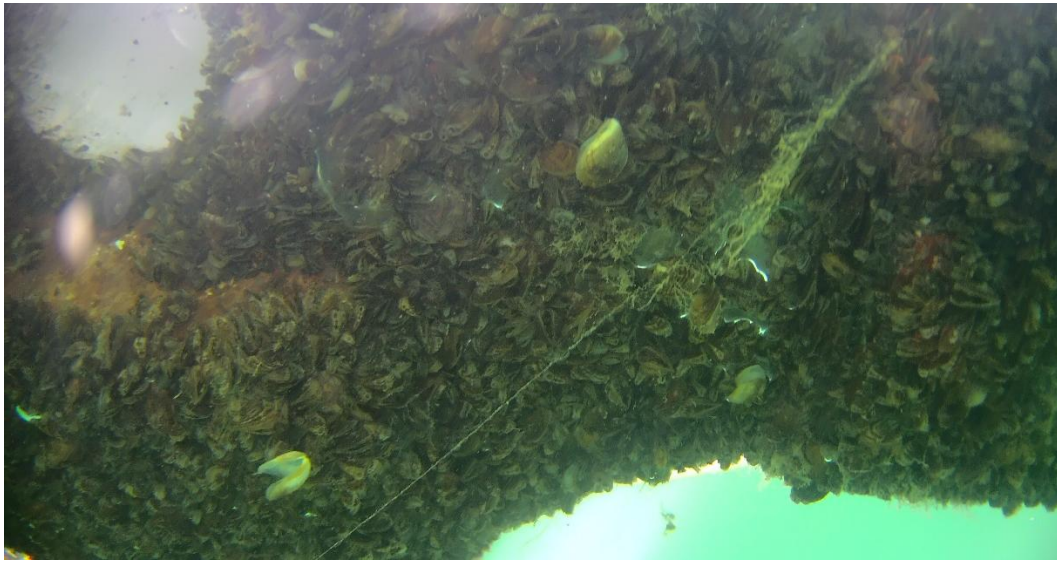
Figure 5-4. Mussels attached to the floaters of the FPV system. Photo taken with Underwater ROV (Deep Trekker 3 ) during a field campaign.
