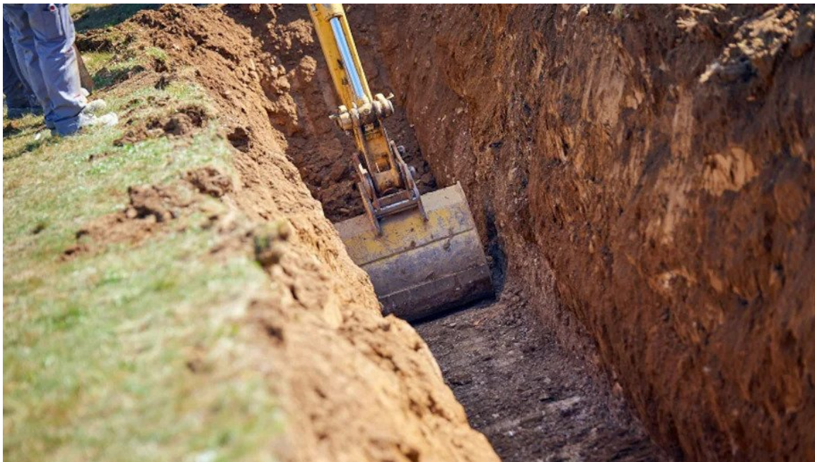
Figure 6.2: The trenching operation using an excavator [170].
