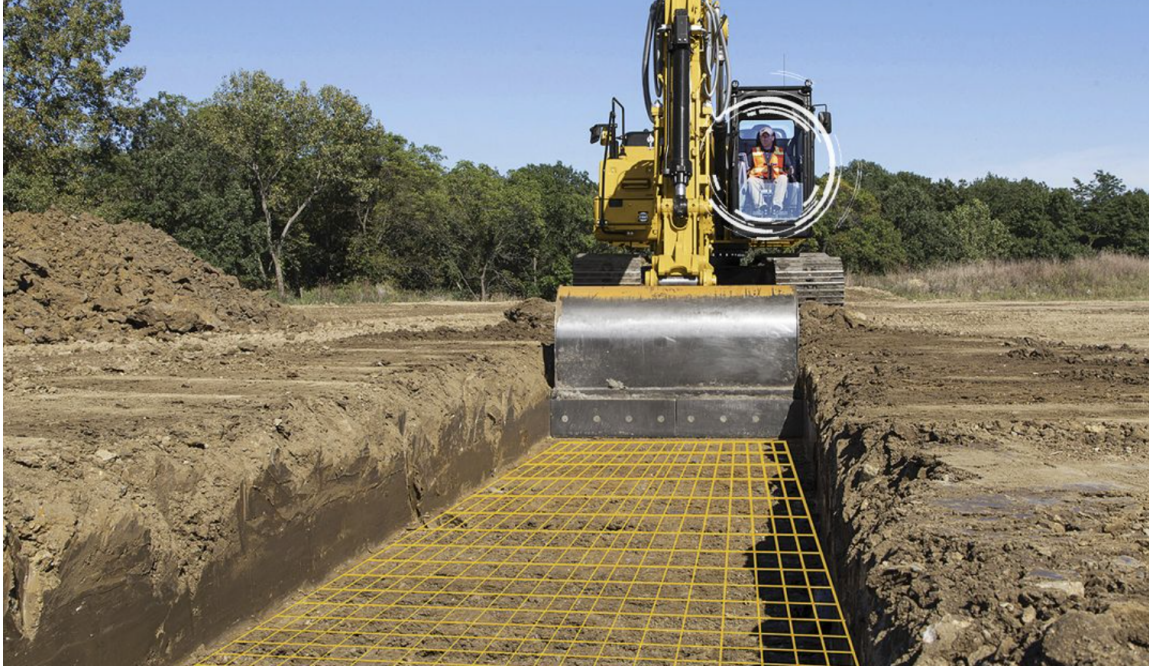
Figure 6.1: The grading operation using an excavator [169].
