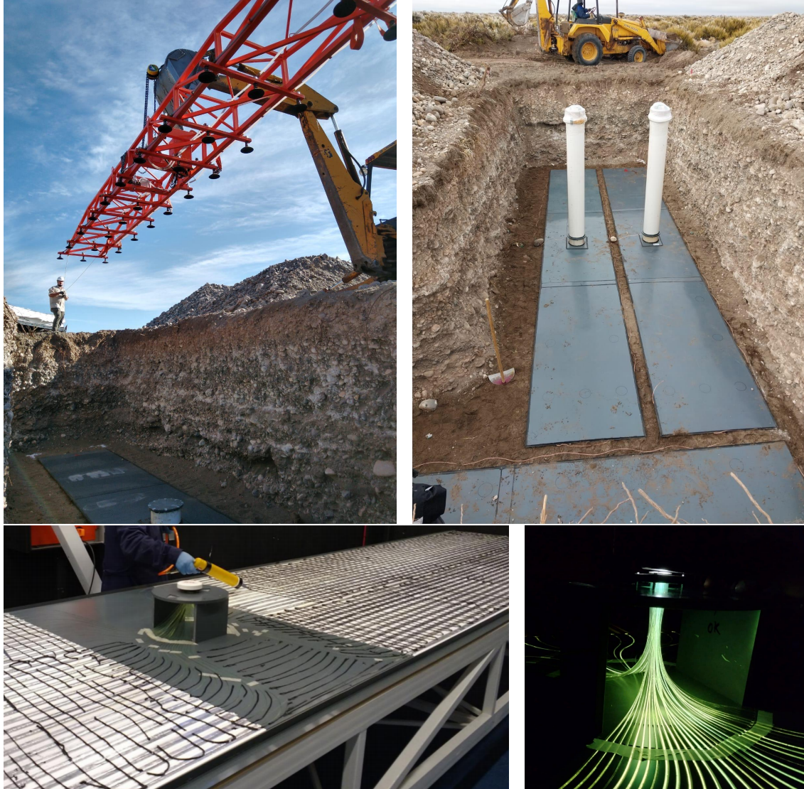
Figure 2.7: (Top) Three modules of 10 \text{ m}^2 deployed in the field. (Bottom) Scintillator module constructed in the assembly building, where we show the scintillation strips (white on the outside) and the WLS optical fibers (green) placed in the cookie.
