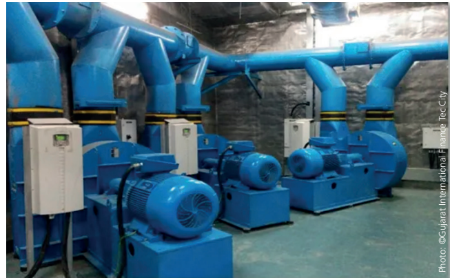
Automated Waste Collection System (AWS) through chute system
