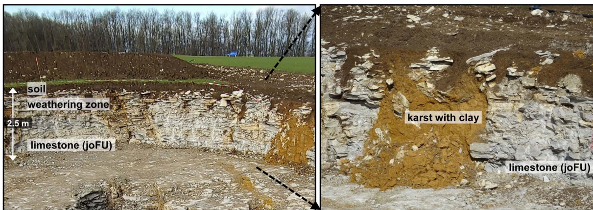
Figure 2. Excavation for the foundation of the southern WT. A thin cover of soil ('Braunerde') is on top of the Jurassic limestone ('Untere Felsenkalkformation, joFU'). The limestone has a weathering zone of varying thickness and karstification with clay fillings. © J. Ritter, KIT-GPI.
