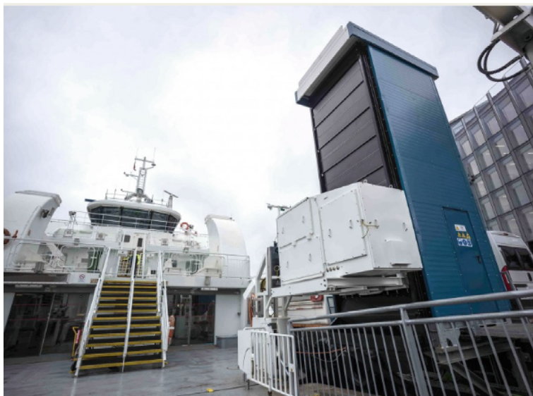
Fig. 3 Automatic plug-in system of the company Cavotec for charging of e-ferries. Source Courtesy Cavotec (2024)
