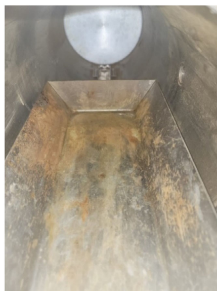
Figure 18. Corroded SS glove box chamber.
