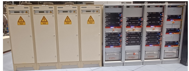
Figure 1: Comparison of old (left) and new (right) quadrupole power supplies. The new units are more compact, modern, and equipped with advanced control systems.
