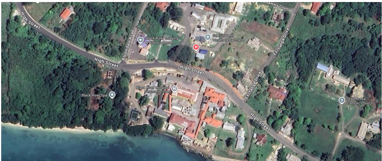
Fig. 14: Satellite image of the Black River Hospital before Hurricane Melissa (Source: https://www.google.de/maps ).
