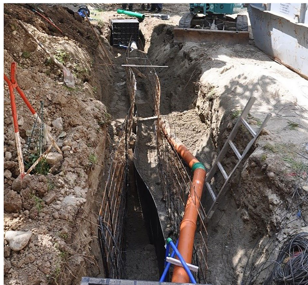
Fig. 3 Installation of the collector, the structural steel mats and the connecting pipes.
