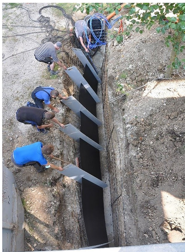
Fig. 2 Installation of the planar collector into the trench.
