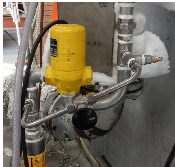
Figure 2. Ammonia fuel supply line equipped with a gas solenoid valve and a bypass, courtesy of the GWI.
