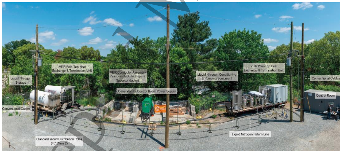
Figure 2. Shows a 30 m single-span suspended version of the O-SCTL demonstrated to understand withstand against outdoor environmental conditions and to utilize commercially available power line structures.
