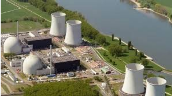
1969 Begin of Biblis A (1300 MWe)
