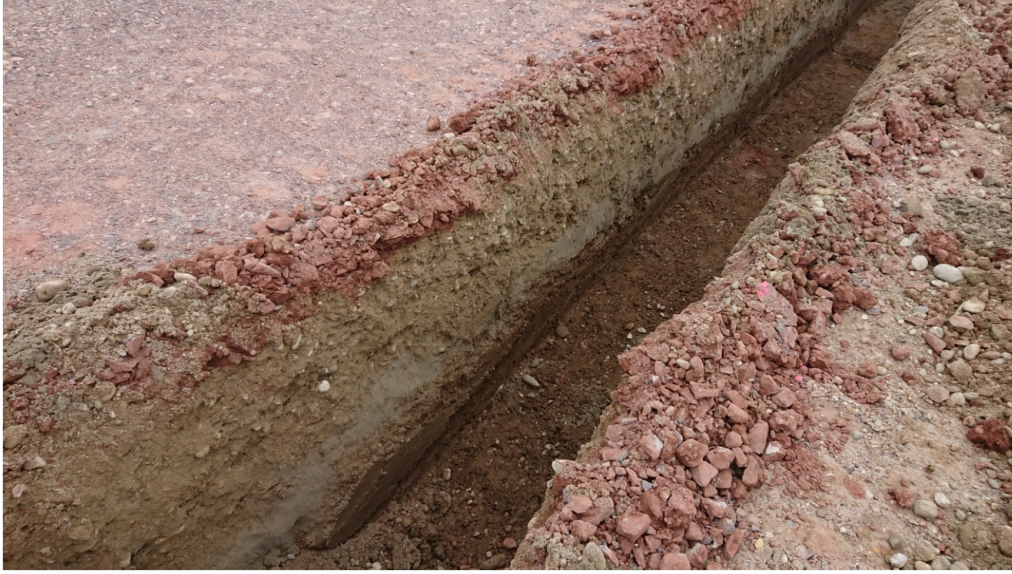
Figure 3.3: Drainage trench at the test site, exposing the near-surface stratigraphy: a thin red-gravel cap over clay-rich soil and underlying coarse gravel with large stones. The trench led to small receiver relocations. Source: Rasho (2025).
