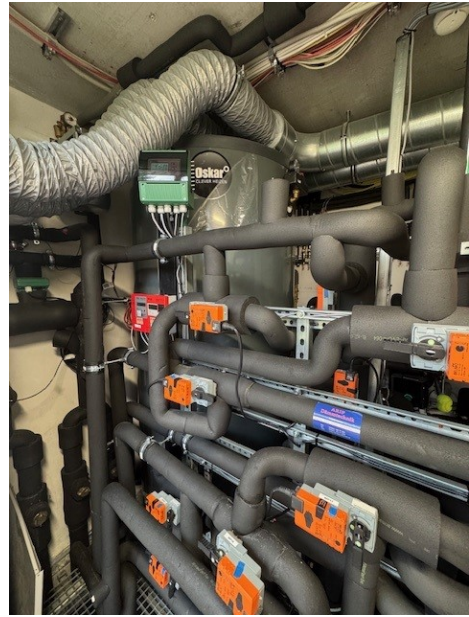
(b) The Oskar hot water storage in the experimental LLEC house
