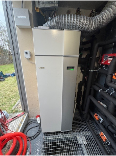
(a) The NIBE heat pump in the experimental LLEC house
