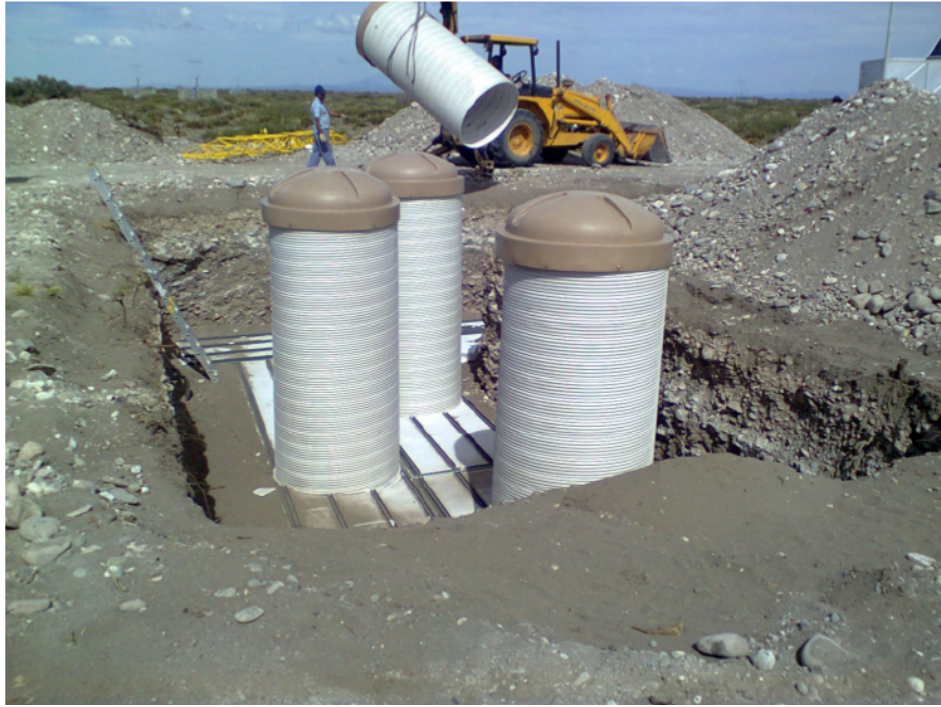
Figure 3.6: Installation of a UMD station with scintillation-based muon counters. Image from [41].
