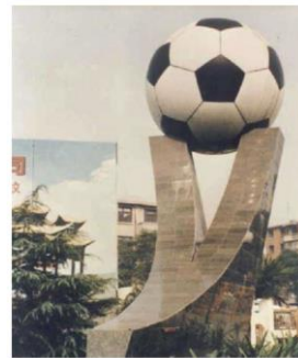
Fig. 1. Hydrobulged steel football of 4000 mm diameter.
