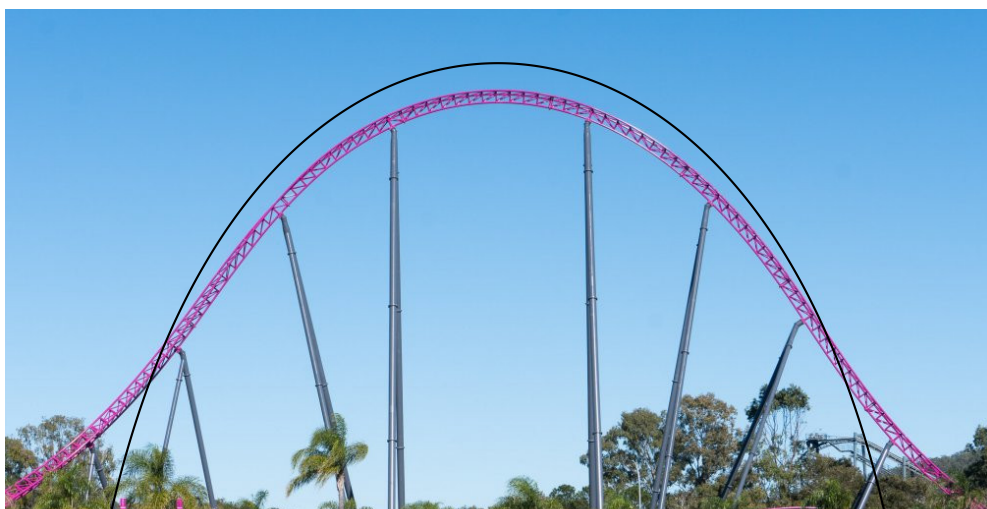
Figure 7.5: Real-world examples of curves of constant acceleration [49; 105].
