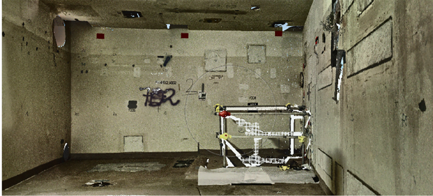
Figure 2: Detailed view of the point cloud of the building structures to be released in Mülheim-Kärlich.
