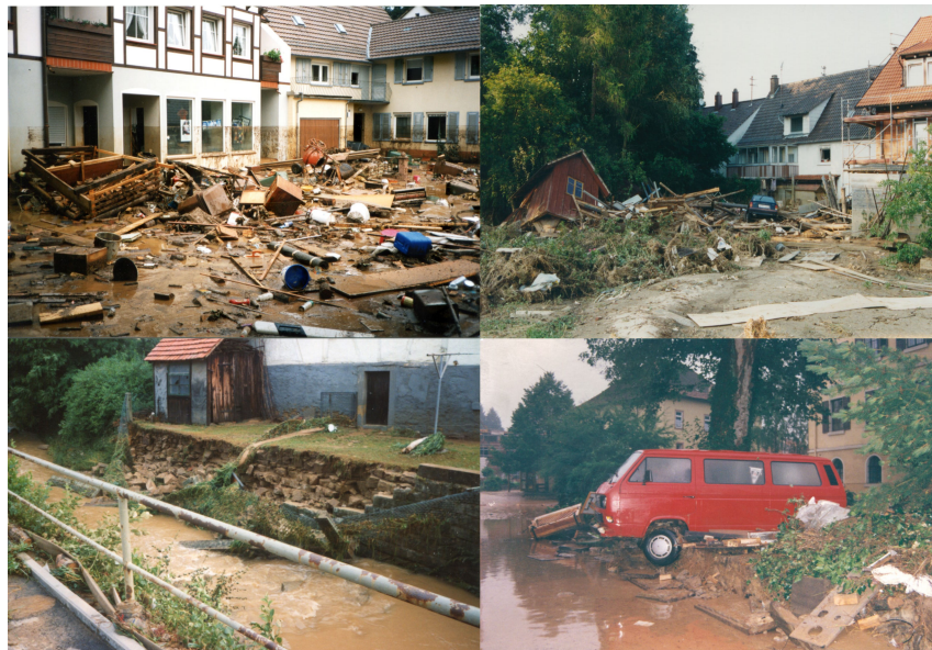
Figure B.8: Aftermath of 27 June 1994 flash floods over the Elsenz-Schwarzbach (Image credit: Archiv Neckarbischofsheim).
