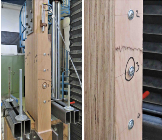
Fig. 3.19: Improper screw insertion: Protruding screw head no. 3.
