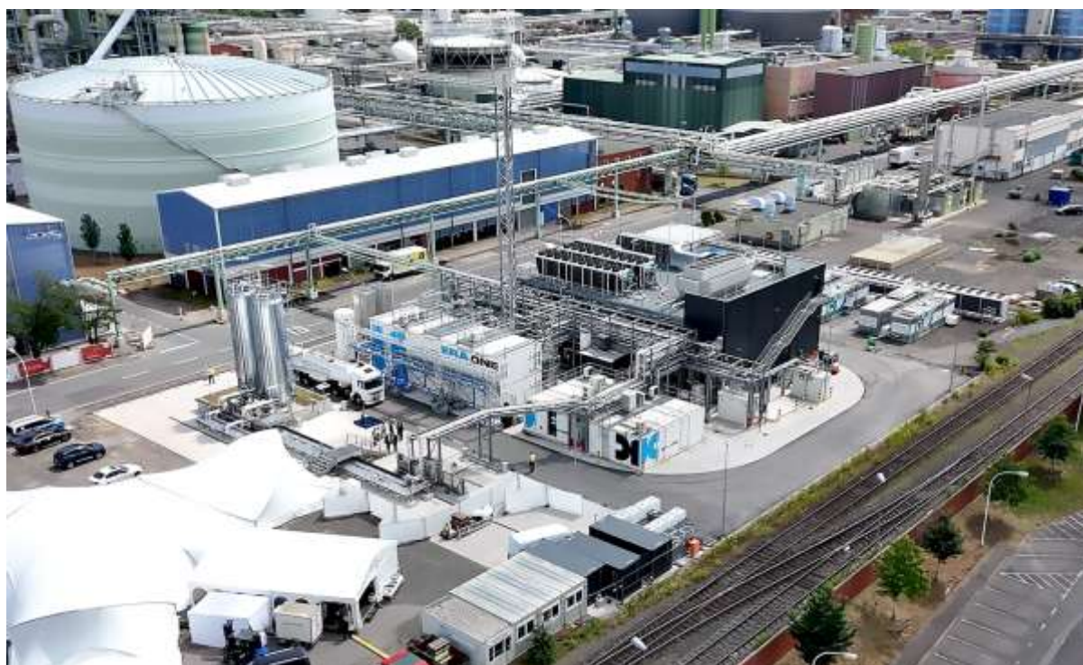
Figure 11.15 Era One site by INERATEC representing the largest production plant for e-fuel in Europe. Green hydrogen and CO 2 from biogenic sources are converted into, amongst others, SAF. Source: INERATEC.
