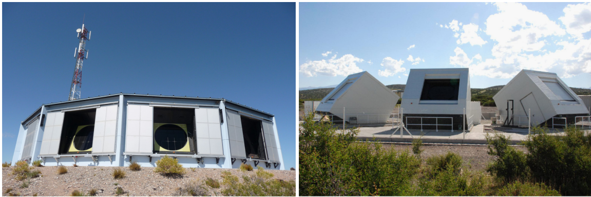
Figure 3.4: (Left) FD building at Los Leones during the day. (Right) Photo of the three HEAT telescopes in tilted mode. The container for DAQ, slow control, and calibration hardware is behind the enclosure of the second telescope. Images taken from Ref [14].
