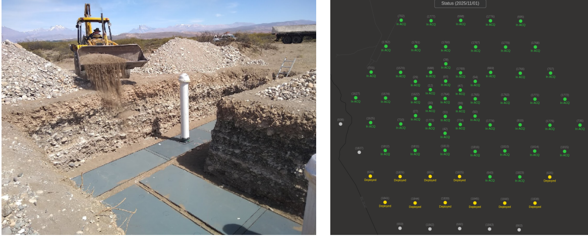
Figure 4.16: Left: Installation of a UMD station during the burial phase at the Malargüe site. The three scintillator modules are positioned in a trench approximately 2.3 m deep, subsequently backfilled with local soil. The vertical conduit houses the optical and power connections to the surface electronics. Right: Deployment status of the UMD as of November 2025. Each circle represents one surface detector station: green markers denote stations in acquisition ( In ACQ ), yellow indicate stations deployed but not yet operational, and grey markers correspond to locations awaiting installation.
